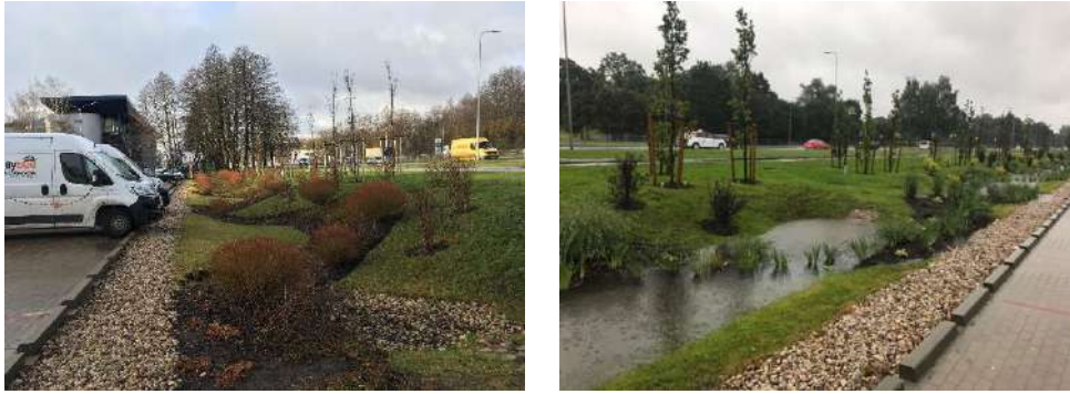
Fig. 2. Bioswale in a parking lot of the SPICE Home shopping centre in Riga city
