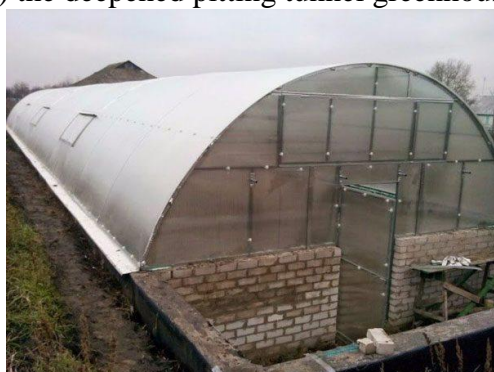
c) the arched or tunnel greenhouse-thermos
